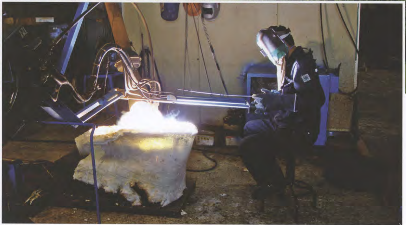
Weld Mold manipulator and arm in operation
